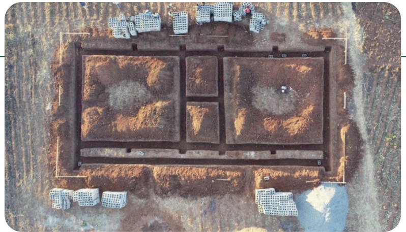
New School Foundations 2026
